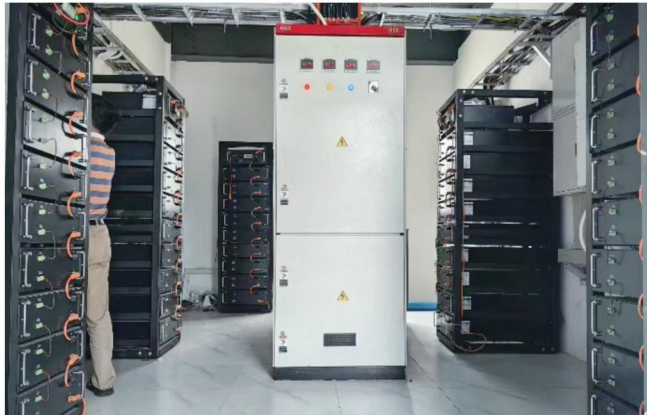
Yangon Textile Factory, Myanmar - 5 High-Voltage Battery Units in Parallel
